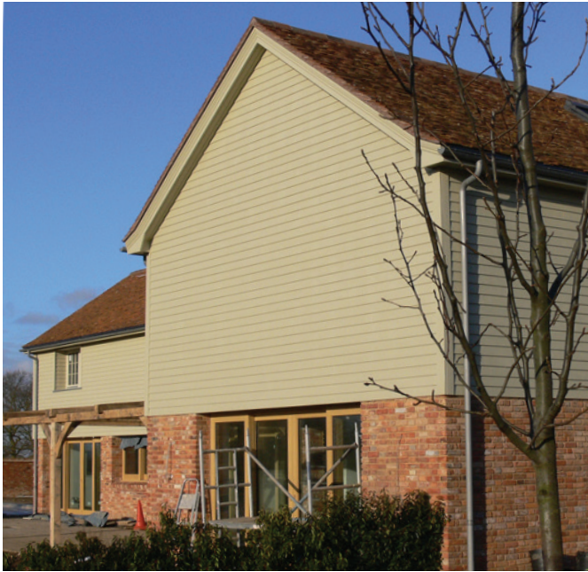
Post occupancy monitoring house in Berkshire
